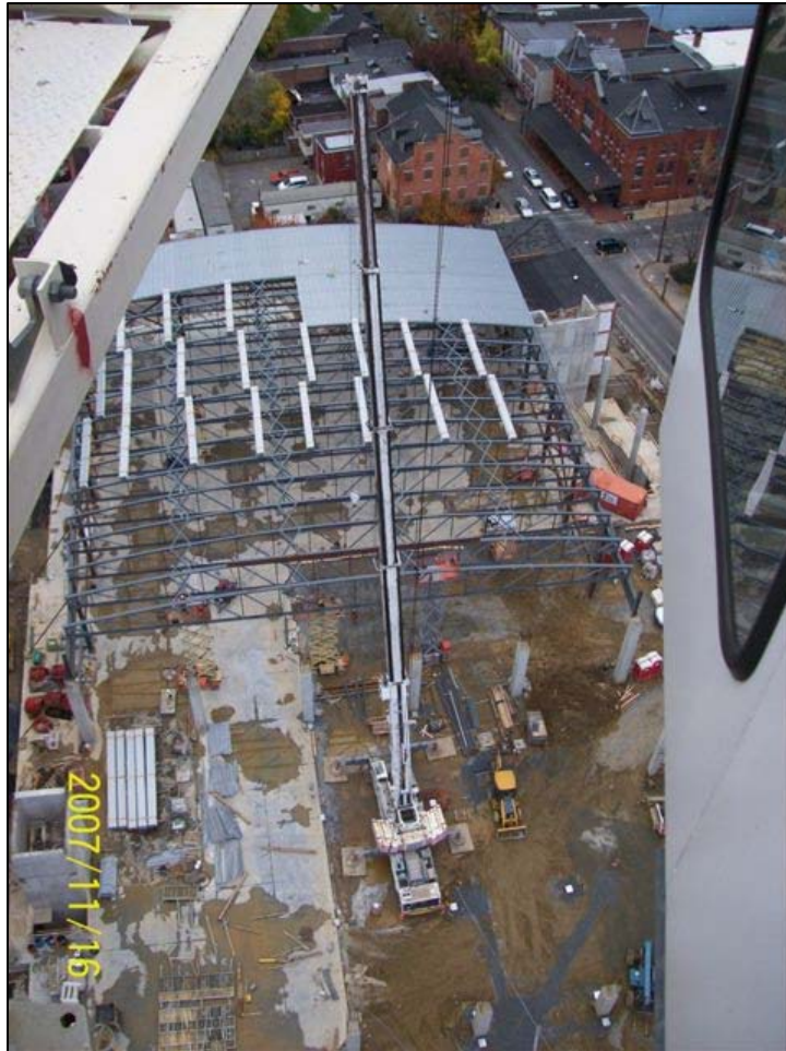
Figure 18 Steel Erection
